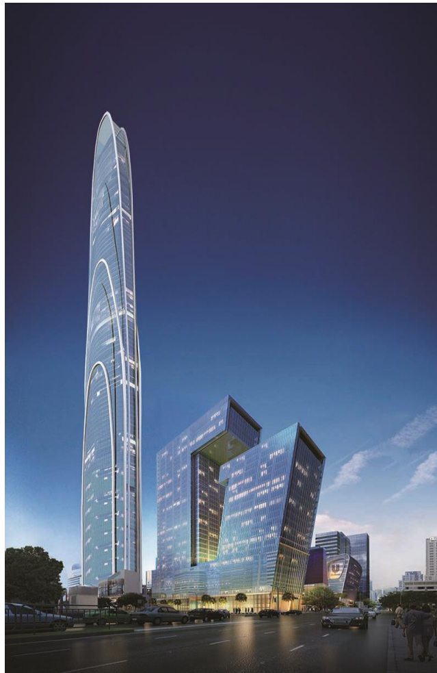
Picture of the G Tower Grand Rama 9 Office Building Project
