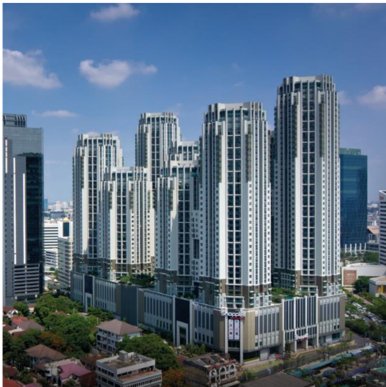
Picture of the Belle Grand Rama 9 Project
